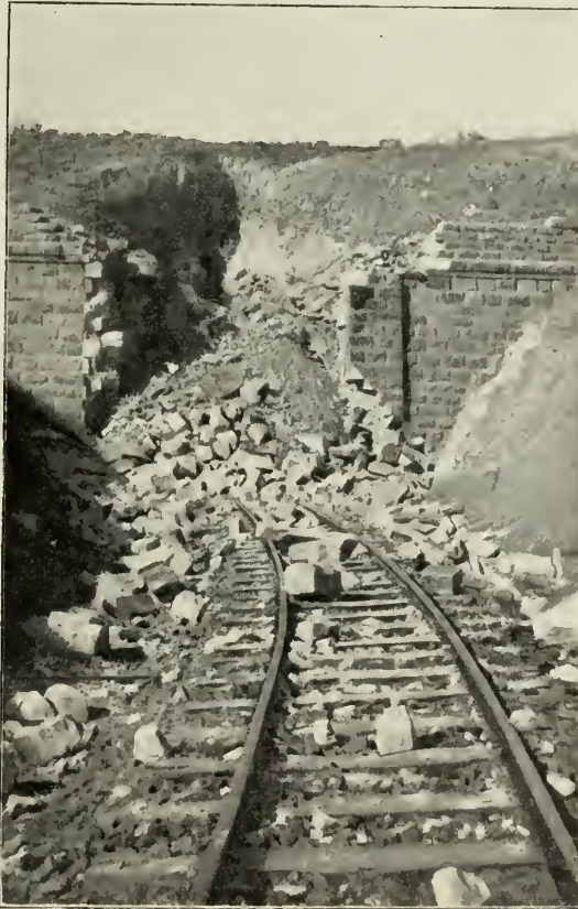
TUNNEL NEAR LAING'S NEK WRECKED BY THE BOERS. North View.
